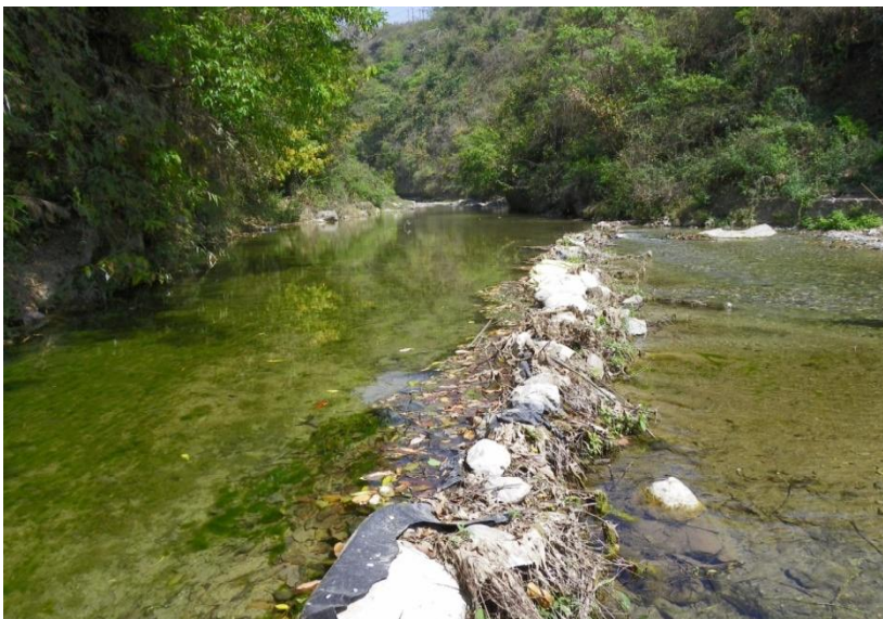
Figure 5: Temporary Alterations of Water Channel in the Middle of the River
